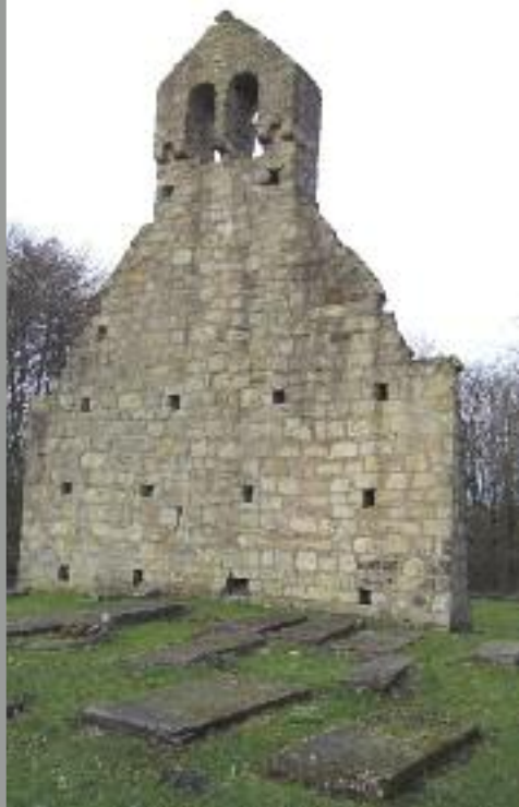
The remaining west gable.
