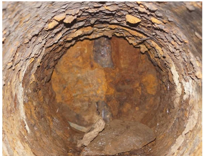
Figure 92. Butterfly valve in inlet pipe.
