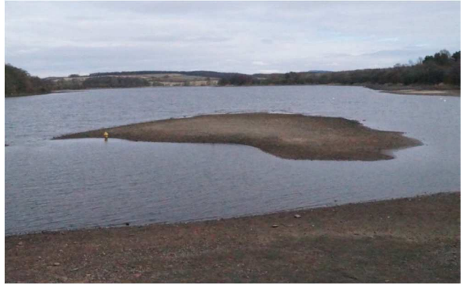
Figure 147. Dam level reduced.
