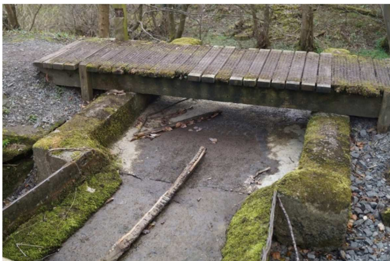
Figure 139. Spillway crosses the lade.
