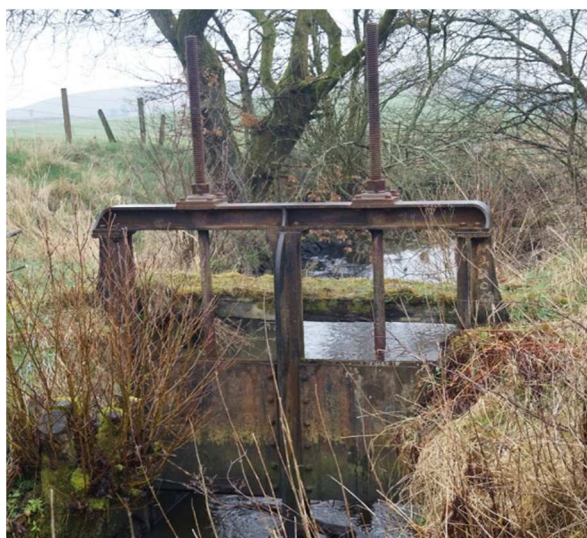
Figure 5. Sluice mechanism.
