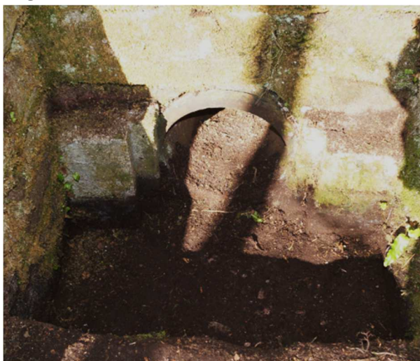
Figure 119. Brick sluice at inlet three.
