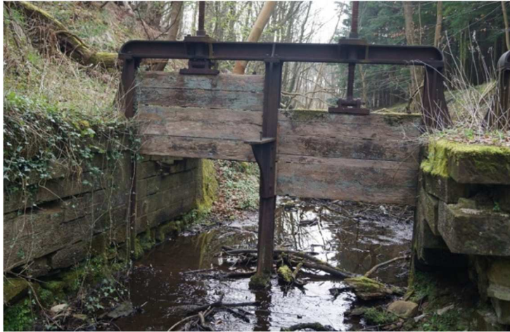
Figure 47. Northern double sluice gates.
