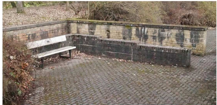
Figure 108. Early 20 th century filter bed walls.
