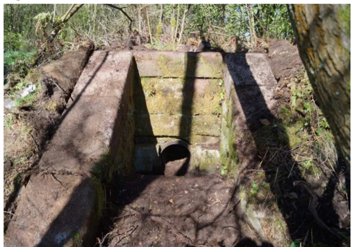
Figure 118. Stone-built inlet number three.
