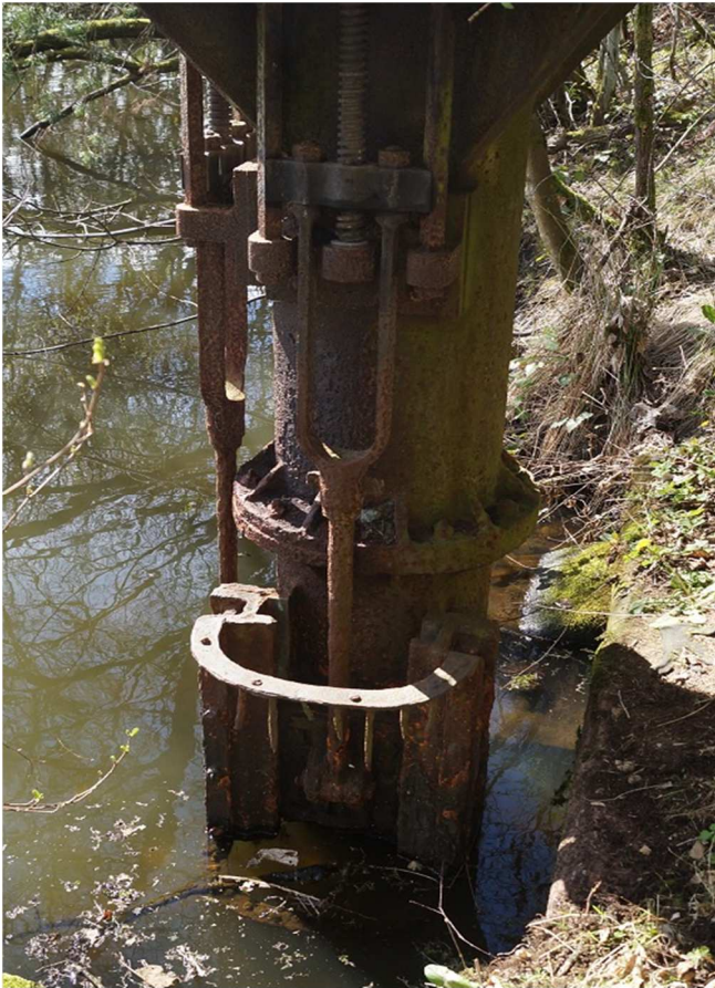
Figure 98. Slide valve screw lifts.
