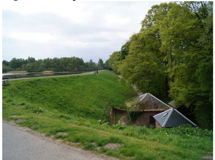
Figure 111. Pump house and water house.
