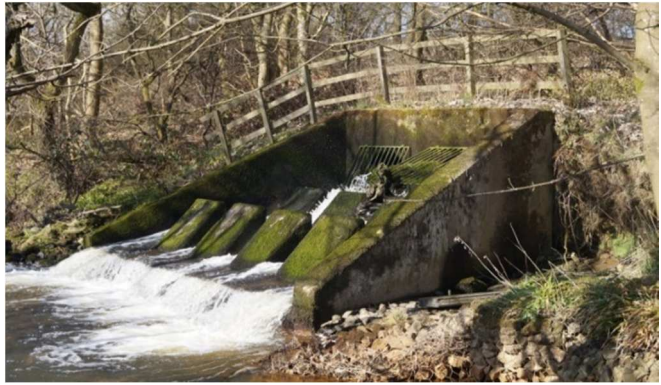
Figure 10. Modern spillway exit.
