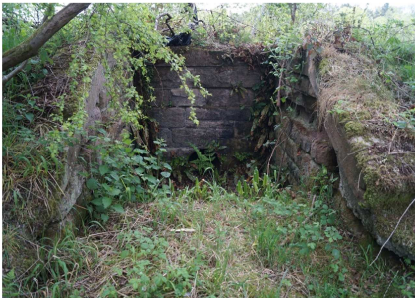
Figure 87. Outlet chamber on the edge of the pond.
