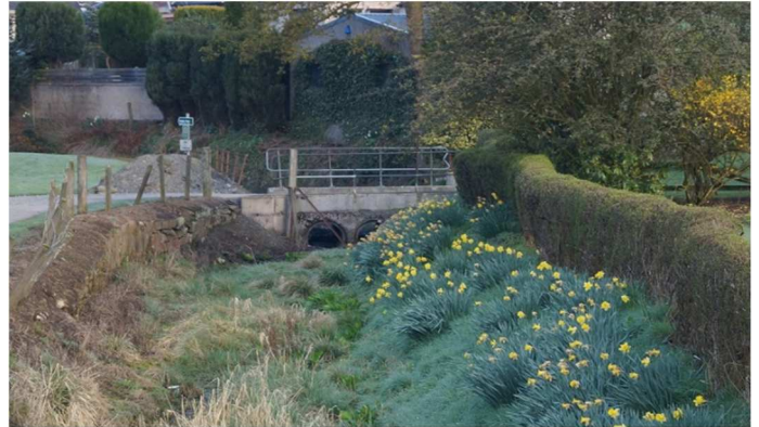
Figure 14. Refurbished iron bridge.
