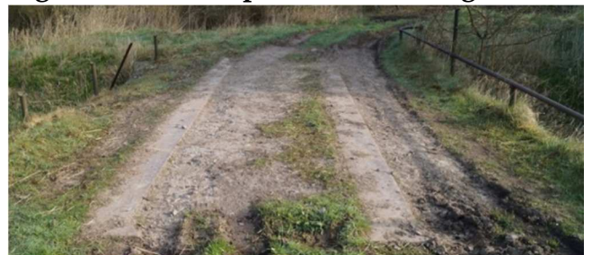
Figure 30. Wheel plate on the bridge.
