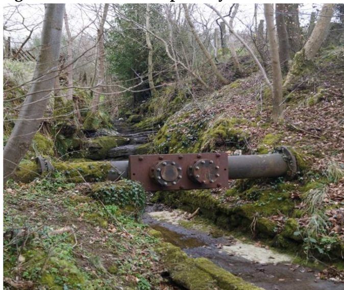
Figure 138. Bottom of spillway channel.
