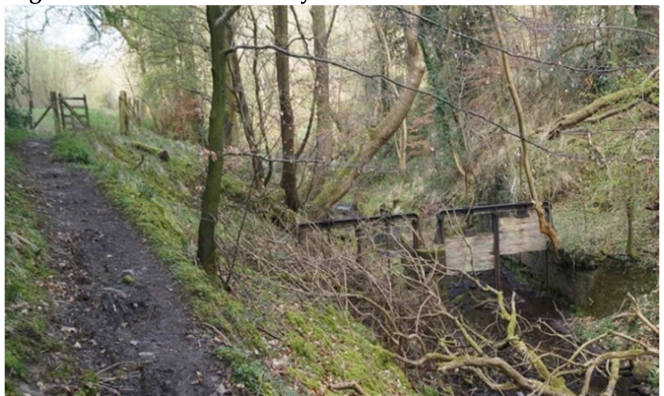
Figure 41. Sluice at the valley end.
