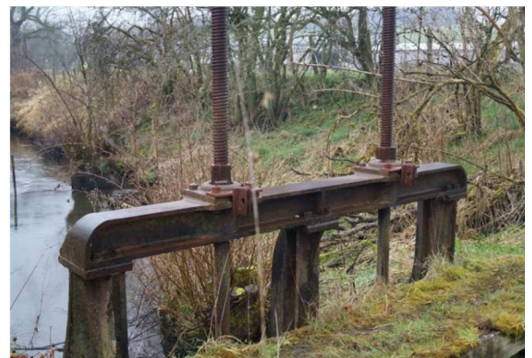
Figure 48. Forestmill sluice gate.
