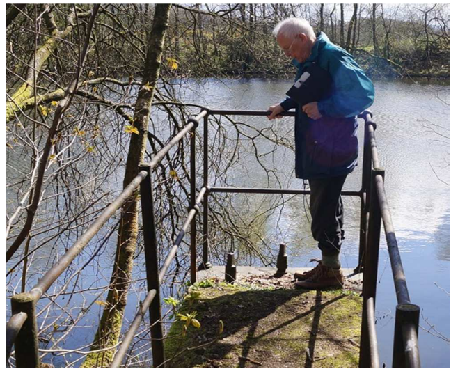
Figure 97. Settling pond outlet tower.
