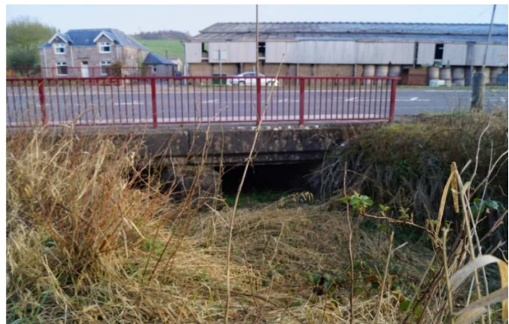
Figure 12. Modern concrete road bridge.
