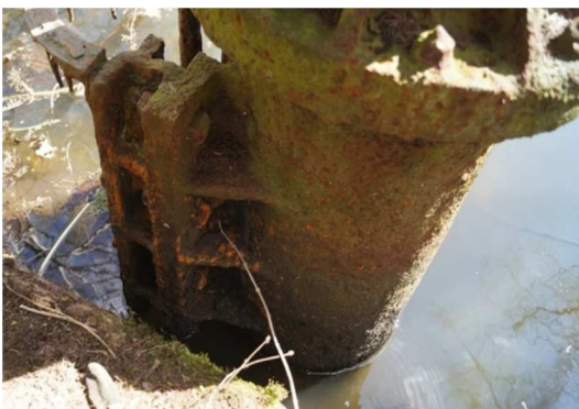
Figure 100. Gate valve side fitting
