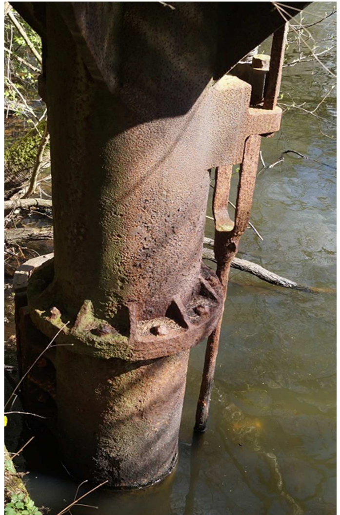
Figure 102. Lower gate valve.
