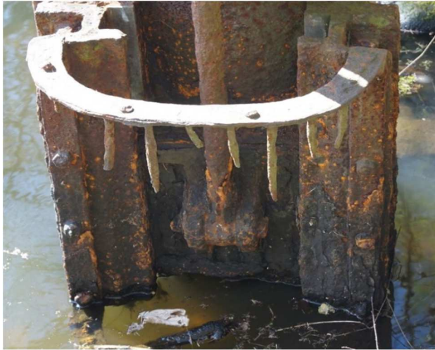
Figure 101. Upper gate valve.
