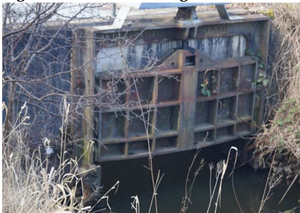
Figure 9. Modern sluice gate.
