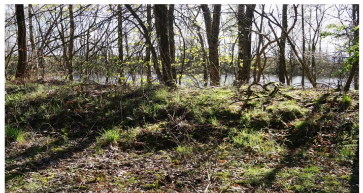
Figure 96. Settling pond embankment.
