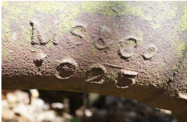
Figure 117. Cast details on pipe.
