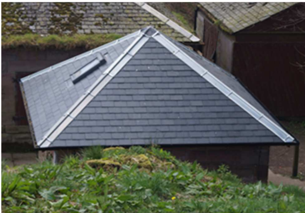
Figure 148. Water house re-roofed.
