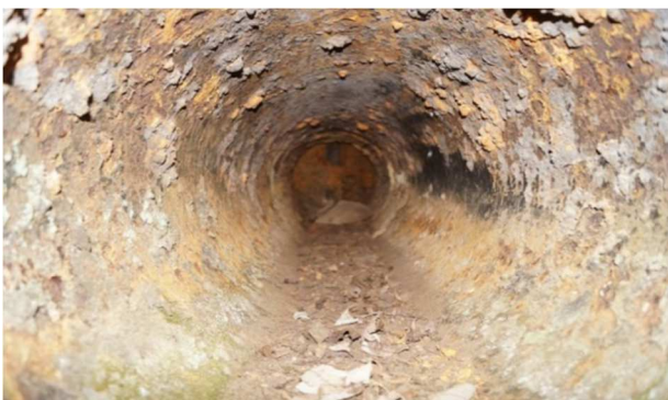
Figure 91. Inside of pipe.
