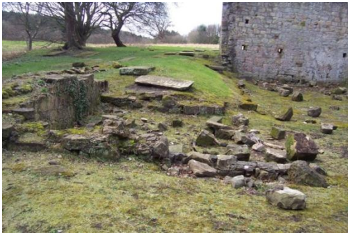
Site before work commenced (by Geoff Bailey)
