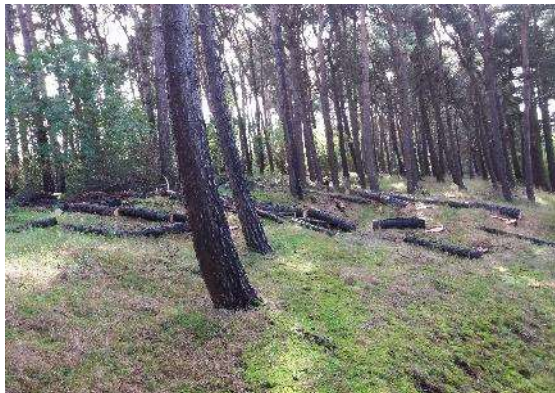
Bothkennar tree felling work, 21 st September 2017
